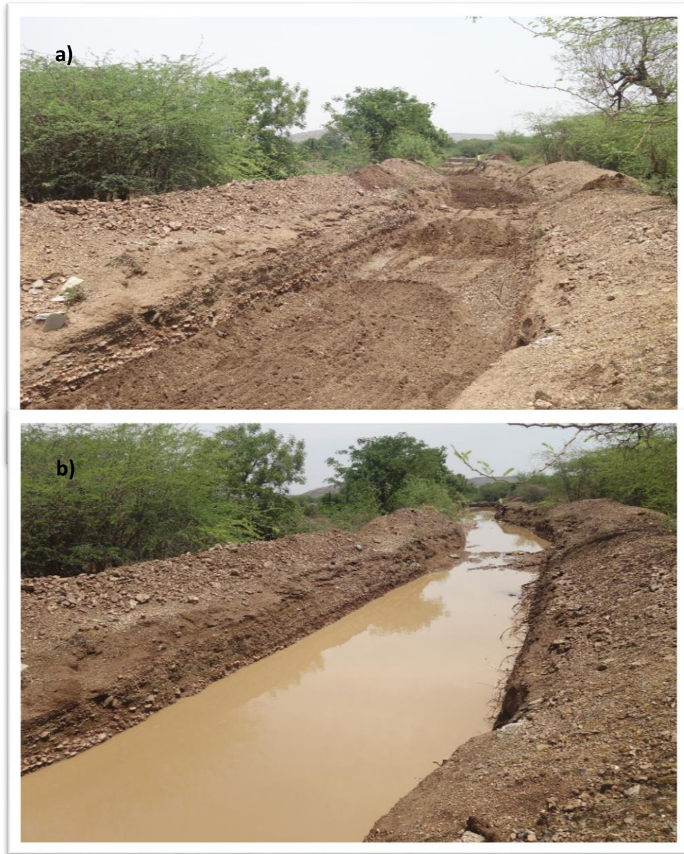
Figure 20. Sunken pits created on a stream in the watershed – a) before rain; and b) after rainfall.
