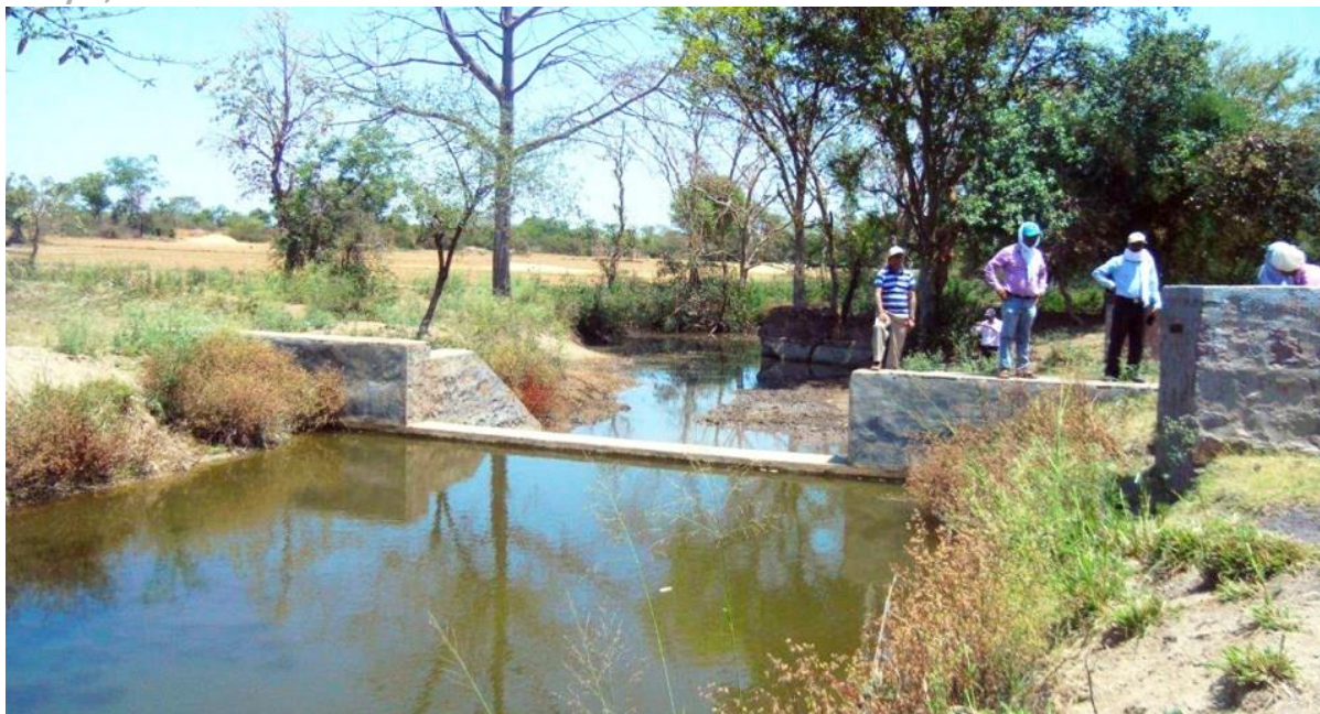
A watershed structure at Parasai-Sindh, Jhansi. Photo: ICRISAT
