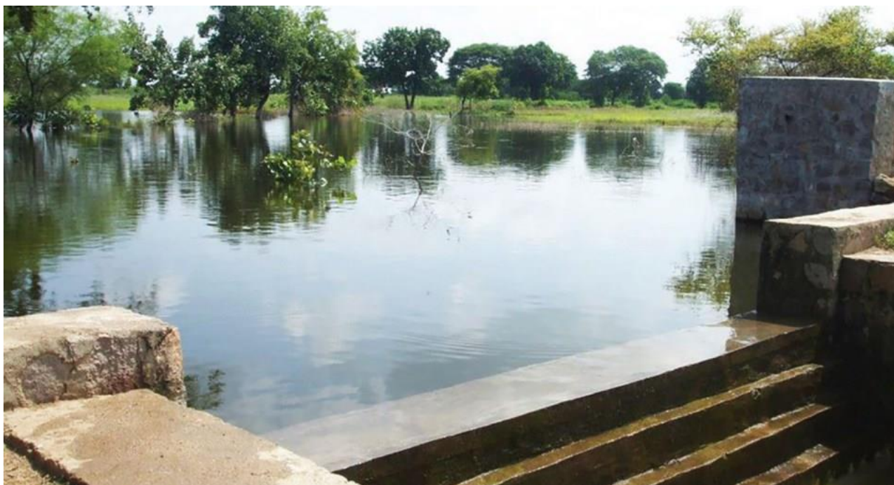
A check dam in Parasai-Sindh watershed in Jhansi, Uttar Pradesh. Photo: Ramesh Singh, CAFRI
