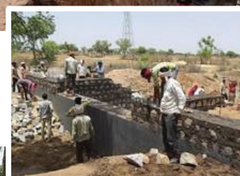
Construction of ensuring checkdam in Baiganur
