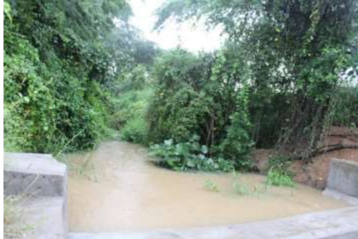
The check dam constructed in Terpole village near Mr N Anji Reddy's farm
