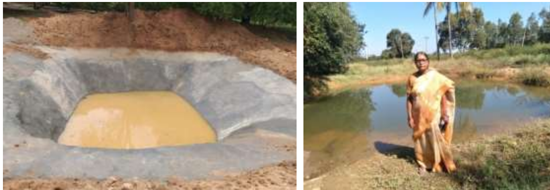
A pond constructed on Ms Sujana's farm in Fasalvadi village.
