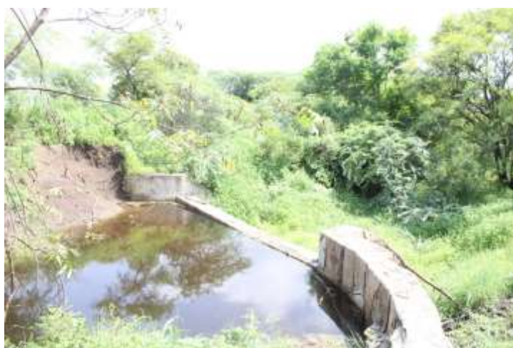
Figure 8. The repaired check dam in Shivampet village near Charminar Brewery.
