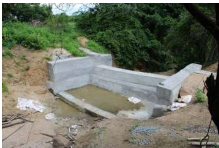
Figure 7. The new check dam constructed in Terpole village near Crown Brewery.
