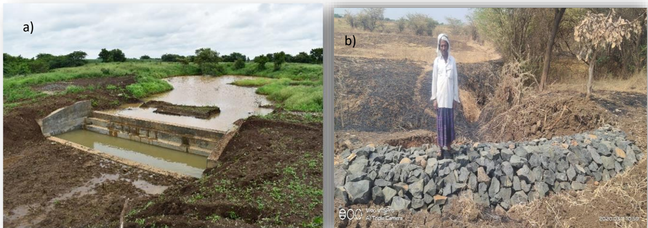
Figure 3. a) Check dam 5 constructed at catchment outlet, 2020, b) Loose boulder structures constructed in the watershed.
