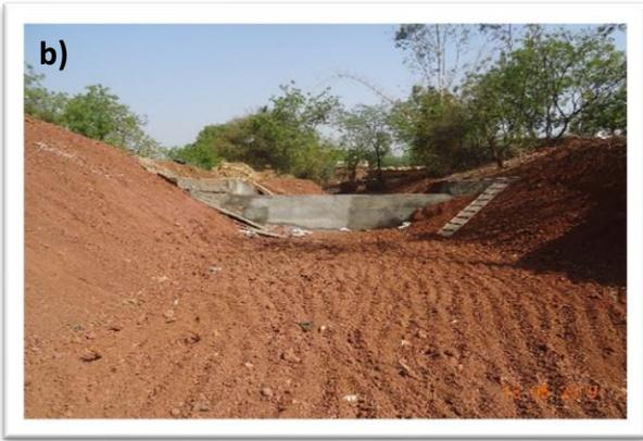
Figure 6. a) Construction of a check dam 4 (in 2019) near to community drinking water supply bore well and b) Stream widening and storage capacity creation at check dam 3 (2019) to harvest rain water.
