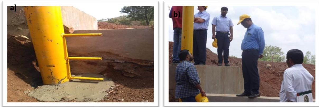
Figure 13. a) Fixing runoff gauging cylinder at check dam no: 3 and b) Explaining runoff gauging procedure to CSR team of Mahindra and Mahindra.
