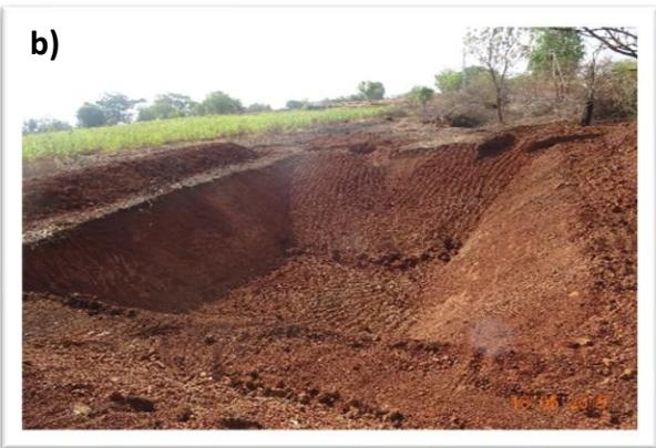
Figure 8. a) Farm pond 1 near to farmer's fields and b) Farm pond 2 near to farmer's fields to harvest rain water during rainy season and utilize as a storage tank during non-rainy season.
