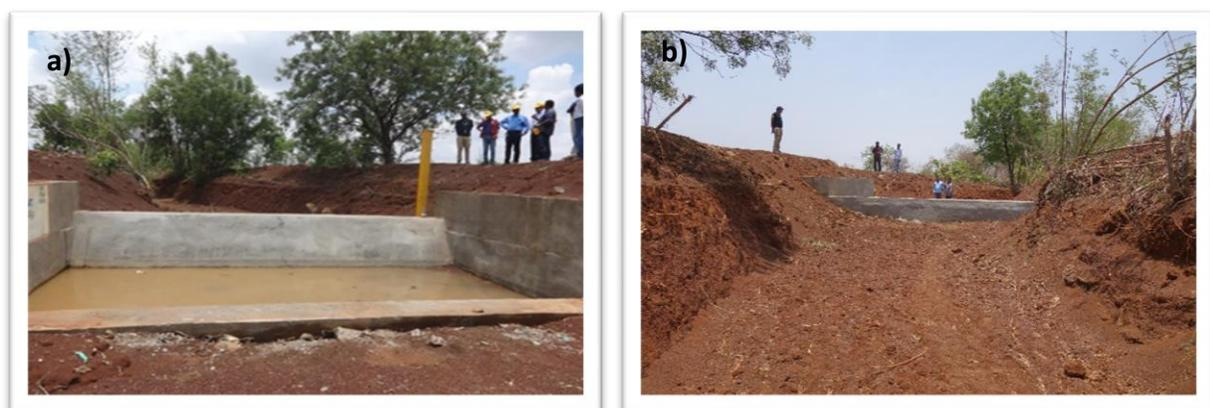
Figure 5. a) Construction of a check dam 3 (in 2019) with runoff gauging station and b) Stream widening and storage capacity creation at check dam 3 (2019).
