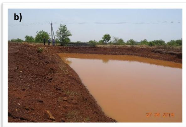
Figure 7. a) Making a mini-percolation tank near to farmer's fields and b) Mini-percolation tank harvesting rainwater during early rains in the month of June 2019.
