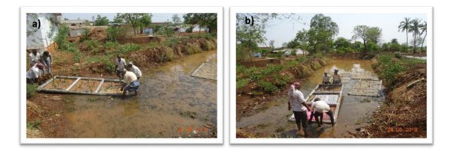
Figure 16. a) Preparing floating wet land b) Setting up floating wetland in the waste water pond in the watershed.
