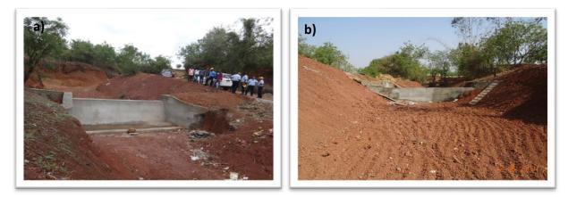
Figure 6. a) Construction of a check dam 4 (in 2019) near to community drinking water supply bore well and b) Stream widening and storage capacity creation at check dam 3 (2019) to harvest rain water.
