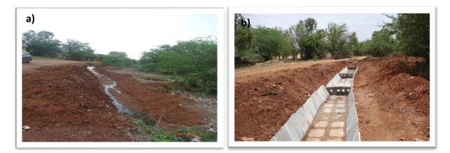
Figure 15. a) Community waste water drainage b) Constructed wet land system on the drainage in the watershed.
