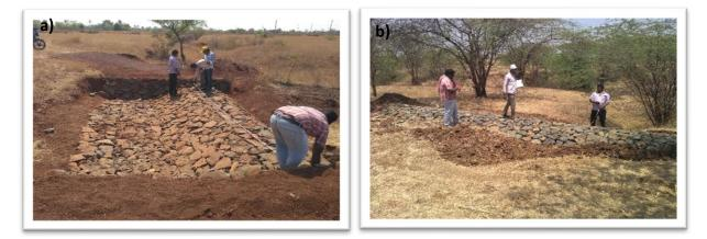
Figure 9. a) Rock fill dam (2 no's) and b) Lose boulder structure (11 no's) constricted in the watershed.
