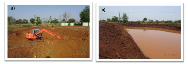
Figure 7. a) Making a mini-percolation tank near to farmer's fields and b) Mini-percolation tank harvesting rainwater during early rains in the month of June 2019.
