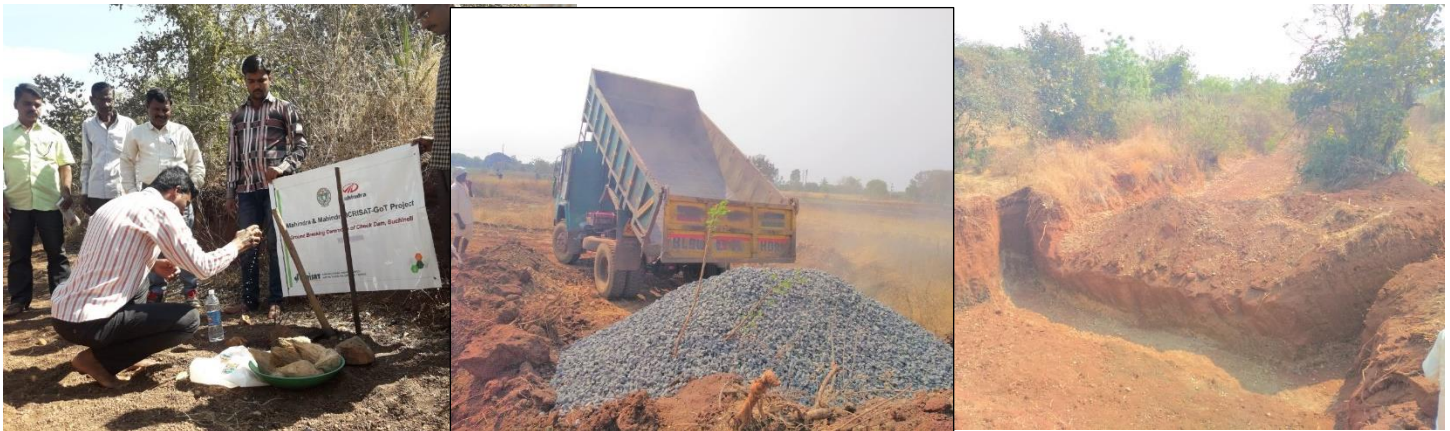
Figure 12. Construction of second check in progress, Buchinelli
