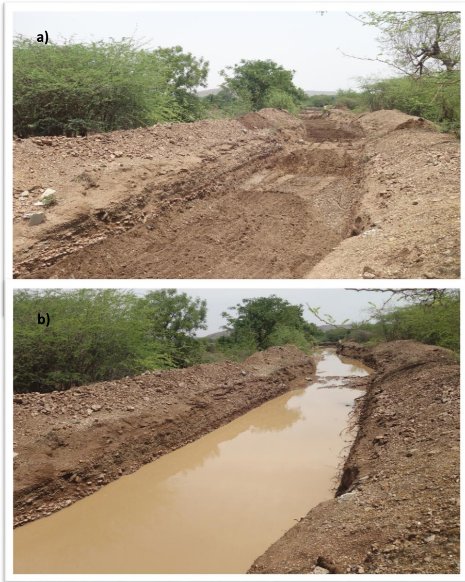
Figure 20. Sunken pits created on a stream in the watershed – a) before rain; and b) after rainfall.
