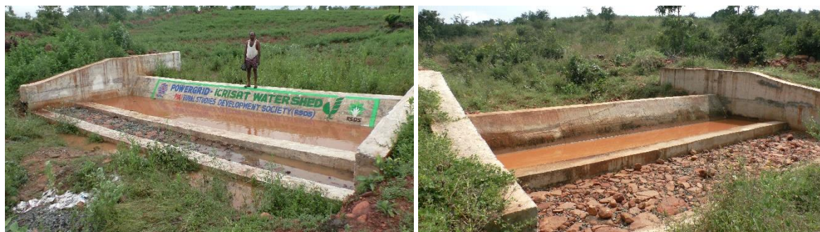
Figure 3. Check dams constructed in (L) Repalle and (R) Muddavaram villages.
