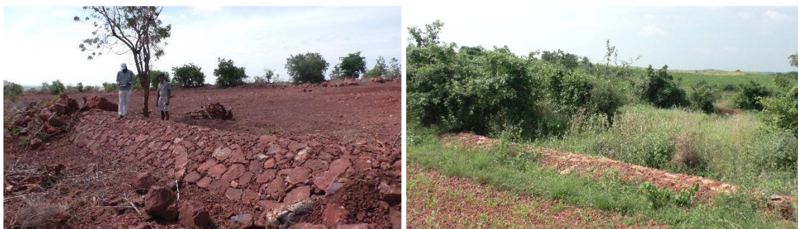
Figure 4. Loose boulder structures constructed in (L) Venkatagiri and (R) Muddavaram villages.
