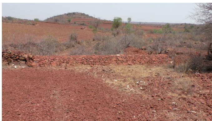
Figure 3. A loose boulder structure constructed in G. Thanda village.
