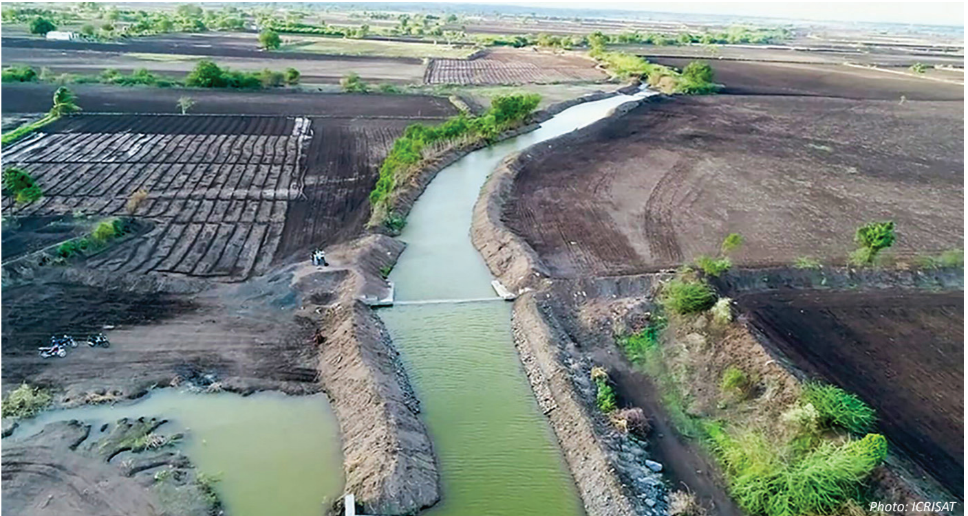
A checkdam constructed in Ukkali to harvest water.
