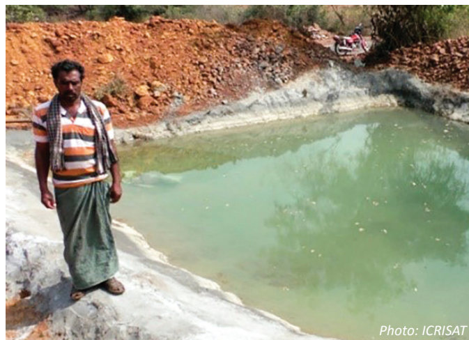
A low-cost cement-lined farm pond that was constructed in Kurnool.
