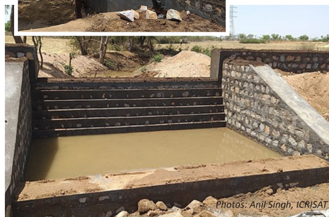
Construction of checkdam in Rajapur village. After completion (below).
