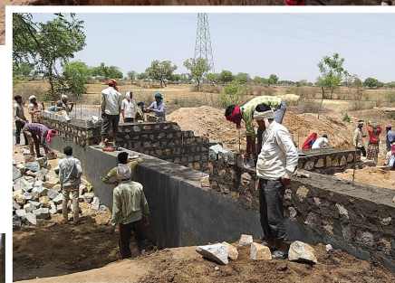
Construction of checkdam in Rajapur village. After completion (below).
