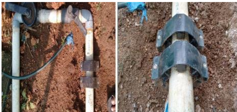
Figure 20: Magnetic water conditioner installed for testing in field at Jumanal village.
