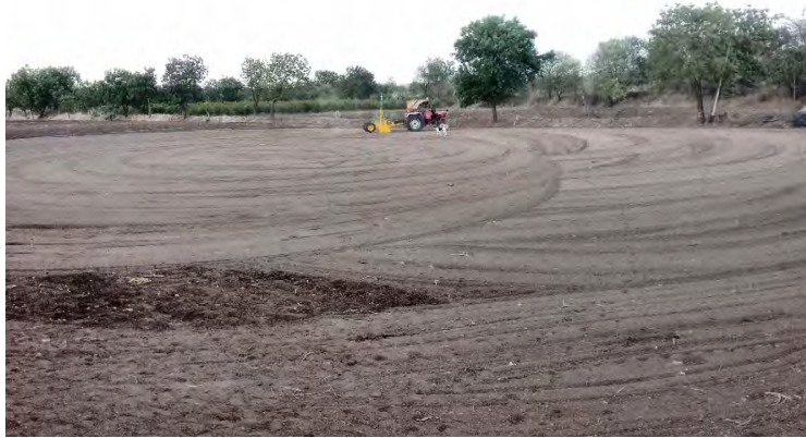
Figure 54. Laser land leveler in operation in Inchageri village
