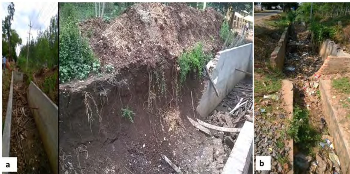
Figure 33. The Lingdahalli constructed wetland site: a) Situation in June 2016; b) Situation in October 2016
