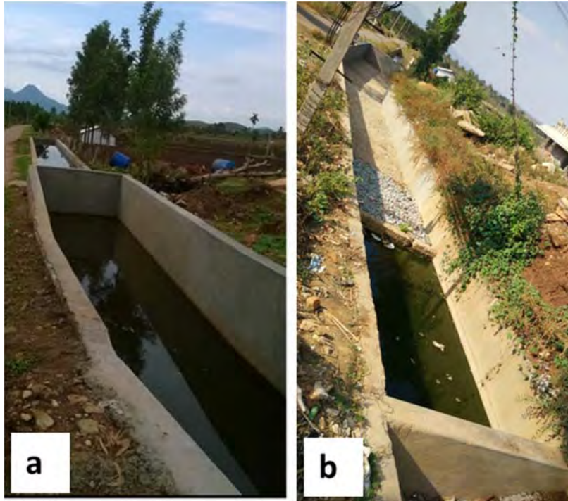
Figure 28. The constructed wetland structures at Sadarahalli a) Situation in June 2016; b) Situation in October 2016
