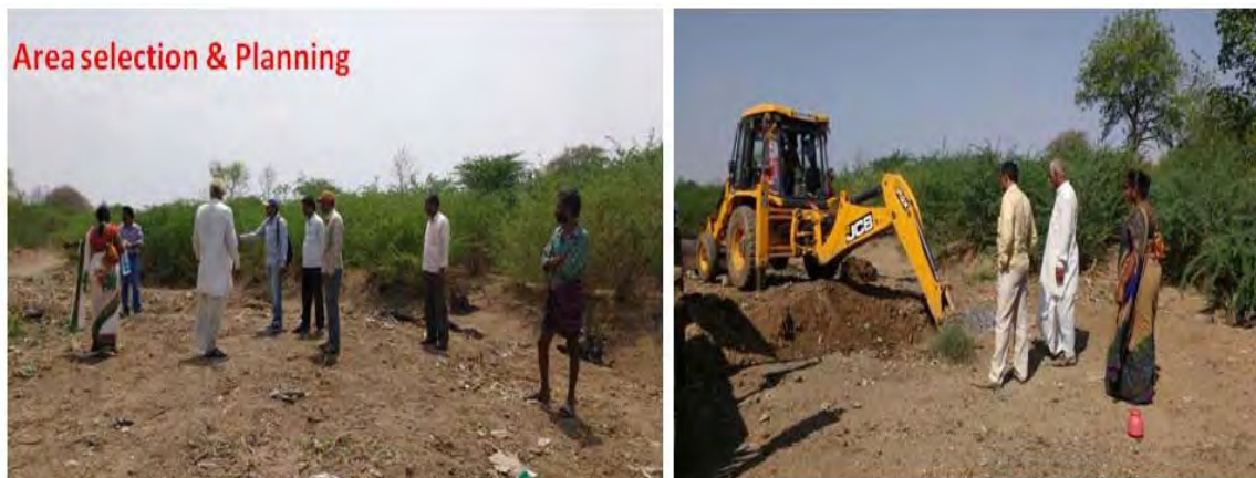
Figure 66. Wet land construction work is in progress in Mulasavagi village
