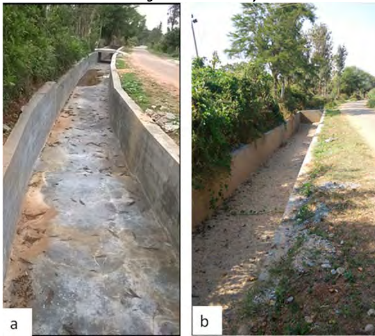
Figure 32. The Lakumanahalli constructed wetland site: a) Situation in June 2016; b) Situation in October 2016
