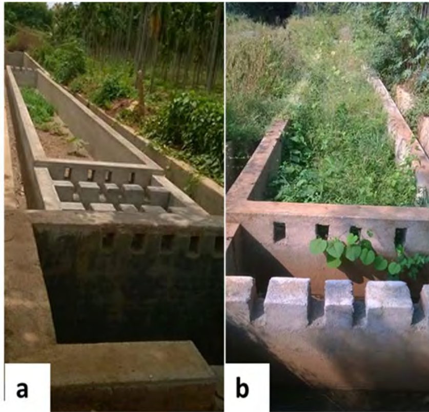
Figure 29. The Udeva constructed wetland: a) Situation in June 2016; b) Situation in October 2016
