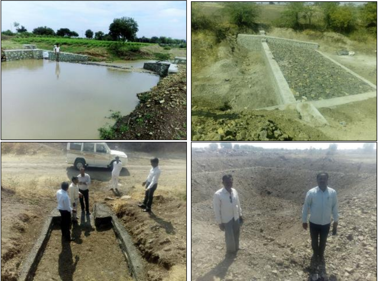
Figure 1. Water harvesting and groundwater recharge structures in Ukkali watershed (from top left clock wise: Check dam, check dam, farm pond and bore well recharge system).
