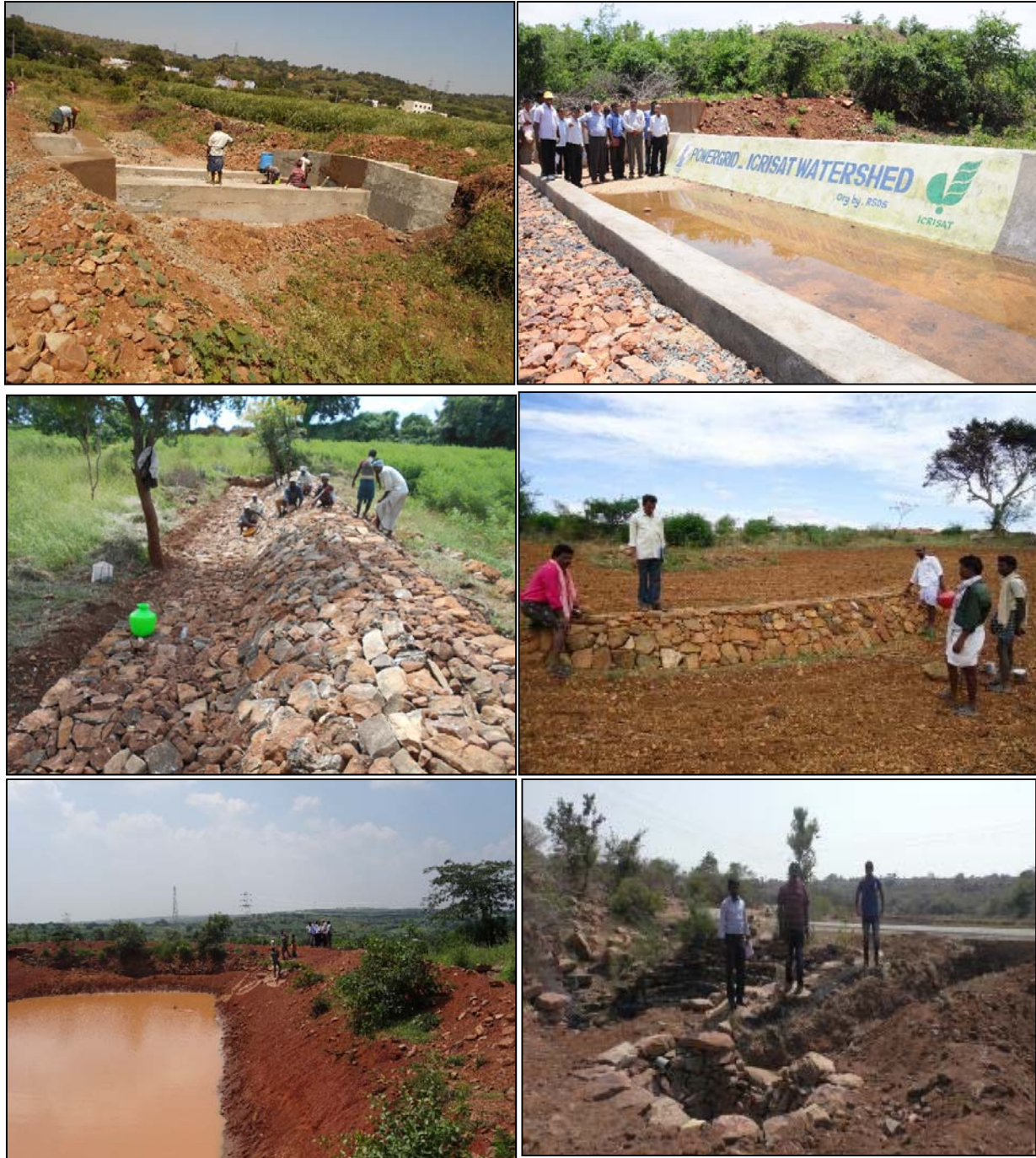
Figure 1. Soil and water conservation structures in POWERGRID-ICRISAT watershed, Bethamcherla, Kurnool district.
