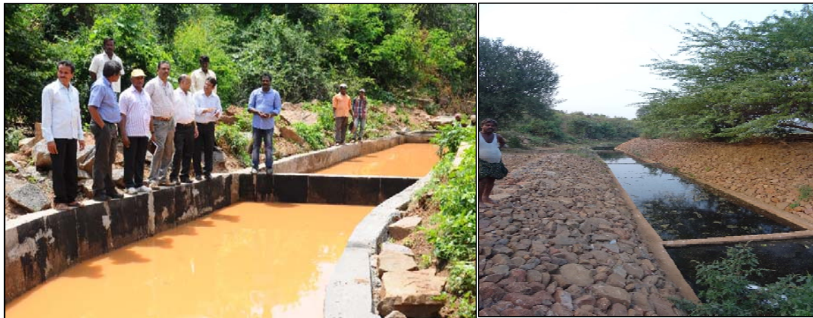
Figure 4. Wastewater treatment unit in M Pendekal, Kurnool.
