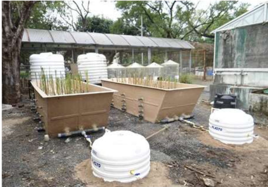
Figure 2-3 Constructed wetland installed at CSIR-NEERI
