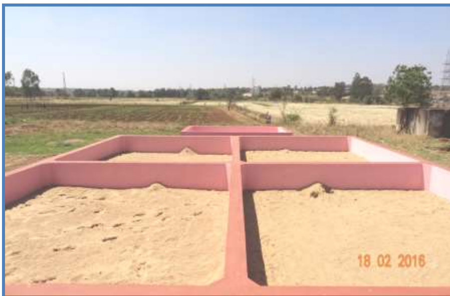
Plate 3. Newly constructed wetland commissioned during 2015-16 at UAS, Dharwad
