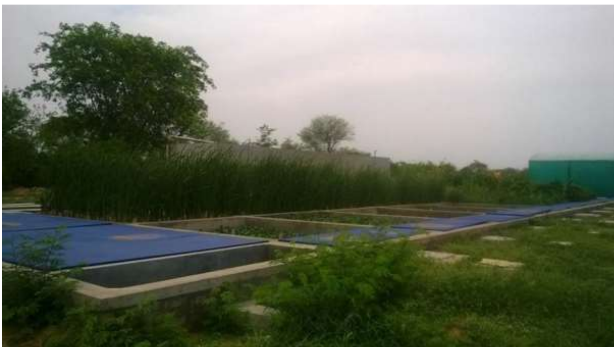
Figure 2-5 View of the all treatment cells of 10 ICRISAT CWs (Photo taken on May 17 2016).
