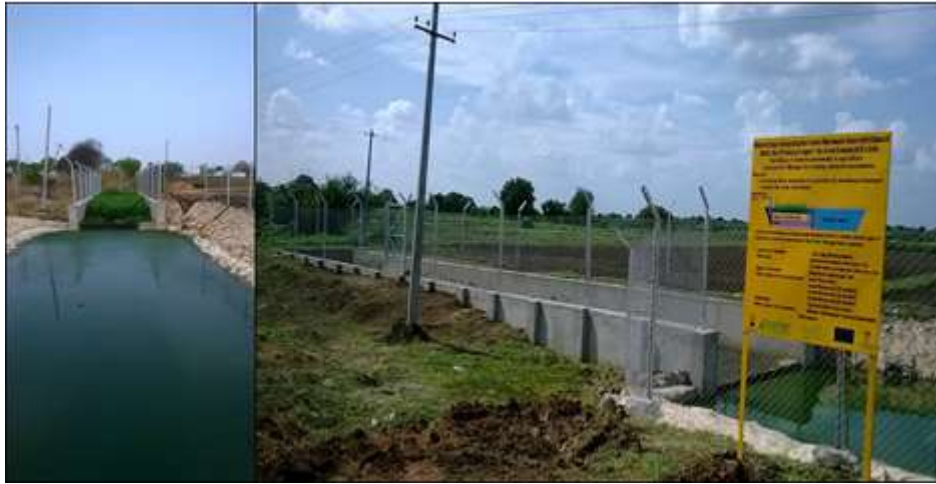
Figure 2-10 CW-2 after stabilization (Oct, 2015)
