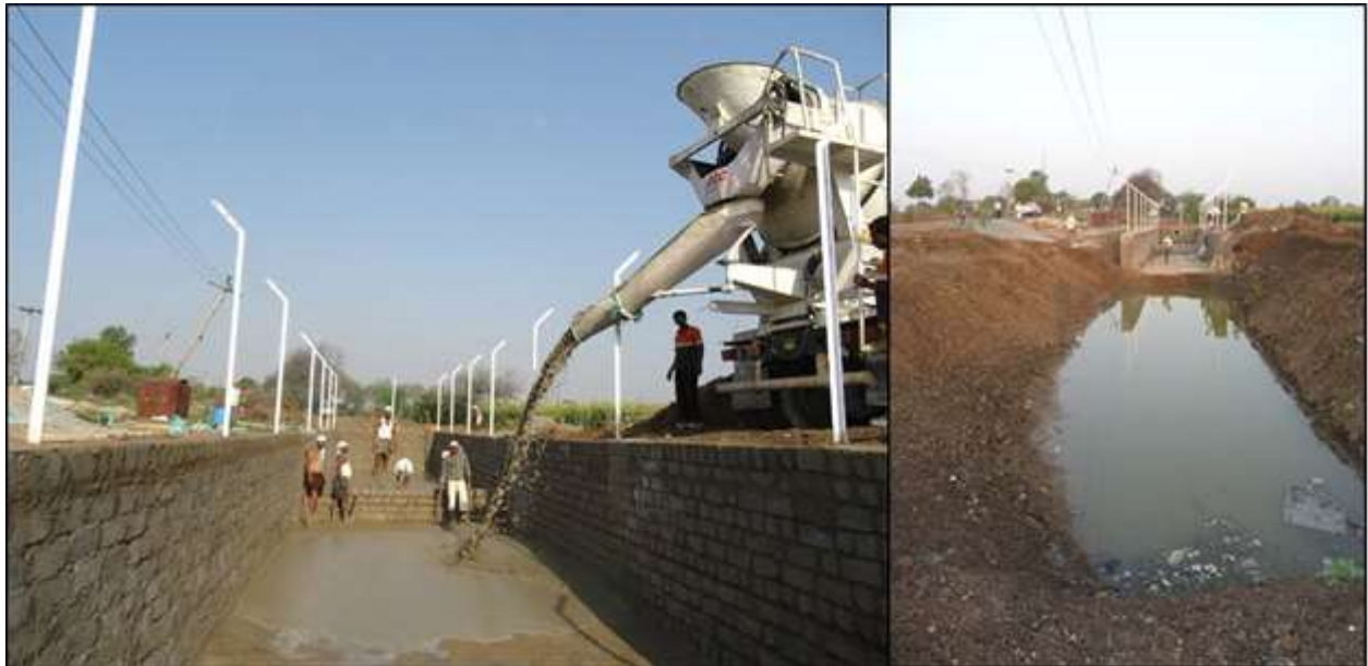
Figure 2-8 Construction phase of CW-2
