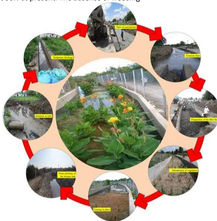
Figure 2-7 Different phases of commissioning of the constructed wetland 1 (CW-1) in Kothapally, Telangana, India.
