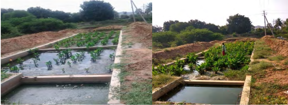
Figure 31. Wastewater treatment units constructed at Chhagattegere in Chikkaballapur district
