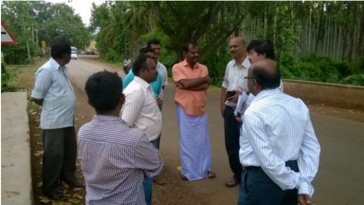
Fig 32: Discussing the poor quality of construction work as well as the land dispute with local leaders and officials at Lingadahalli (Tarikere, Chikmagalur) site.
