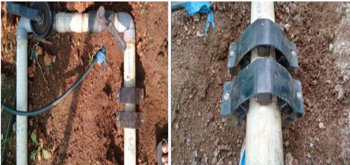
Figure 97. Magnetic water conditioner installed for testing in field, jumanal village.
