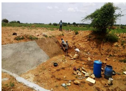
Figure 6.1.1.5: A Farm pond under construction
