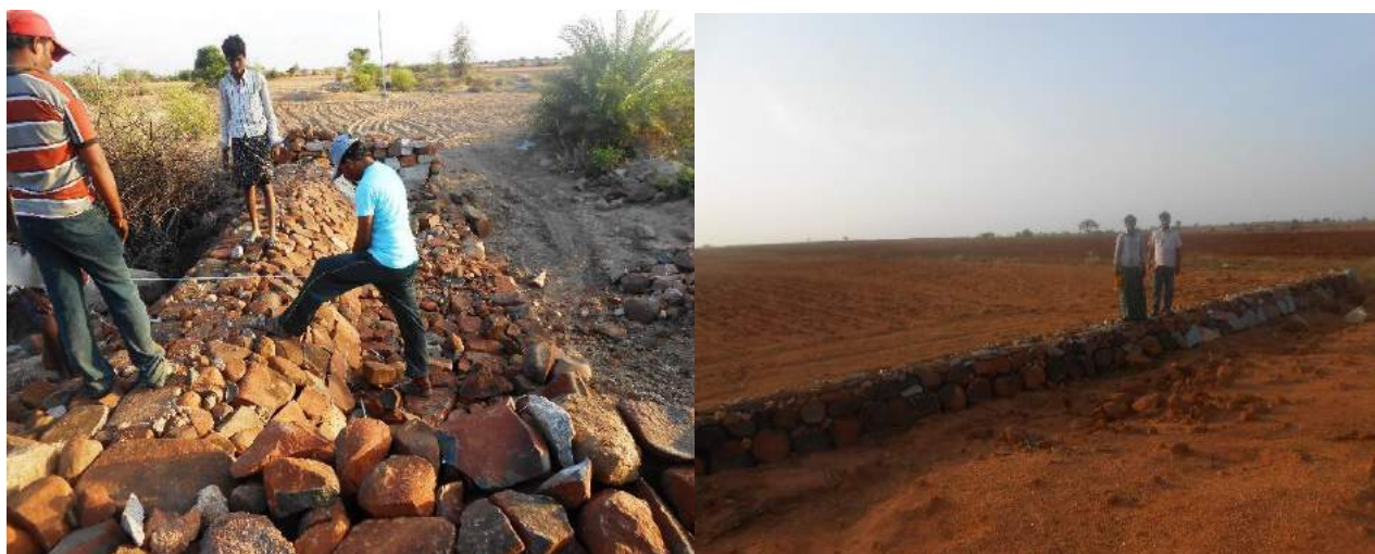
Figure 4.1.7.8. Rock fill dams and loose boulder structures for soil and water conservation
