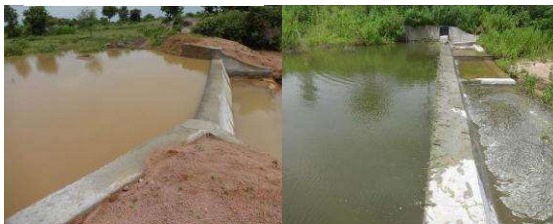
Figure 6. Masonry checkdams with stored runoff water in Sulthanpur (left) and Fasalvadi (right) villages
