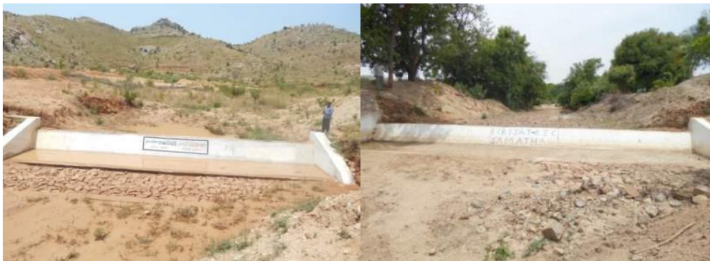
Check dams (Settipalli and Gonipeta)
