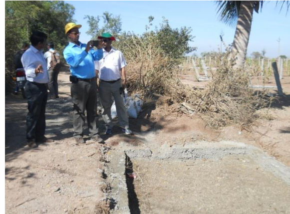
Borewell recharge pit
