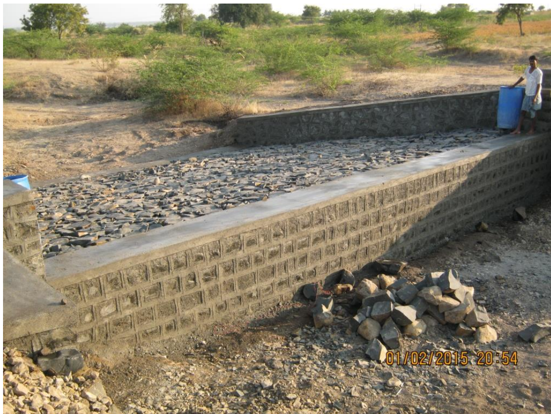
Masonry check dam
