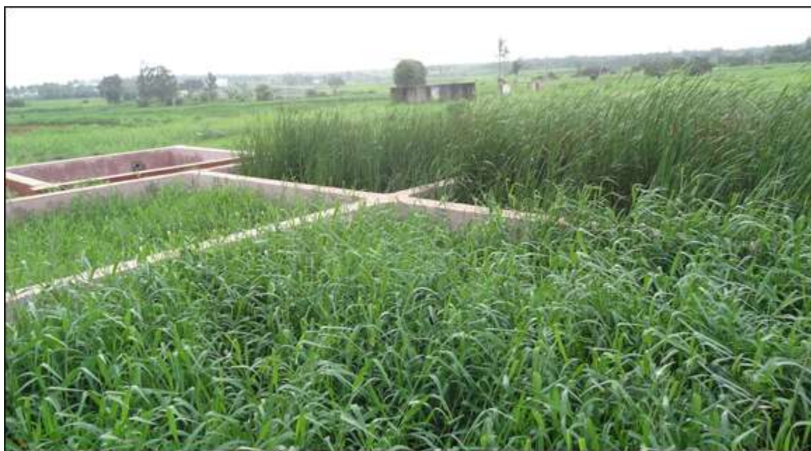
Figure 2-16. Constructed wetland at UAS, Dharwad for treating domestic wastewater
