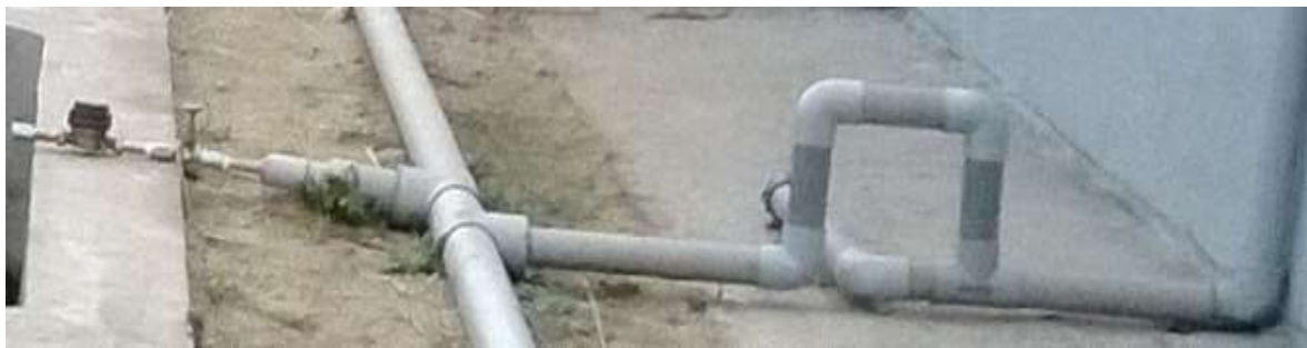
Figure 2-9. The U-bend and sludge drain at the wetland inlet
