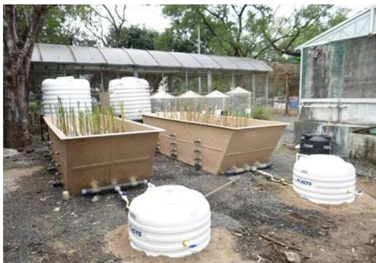
Figure 2-7. Pilot scale demonstration of ECWs for the treatment of domestic wastewater installed at CSIR-NEERI campus, Nagpur
