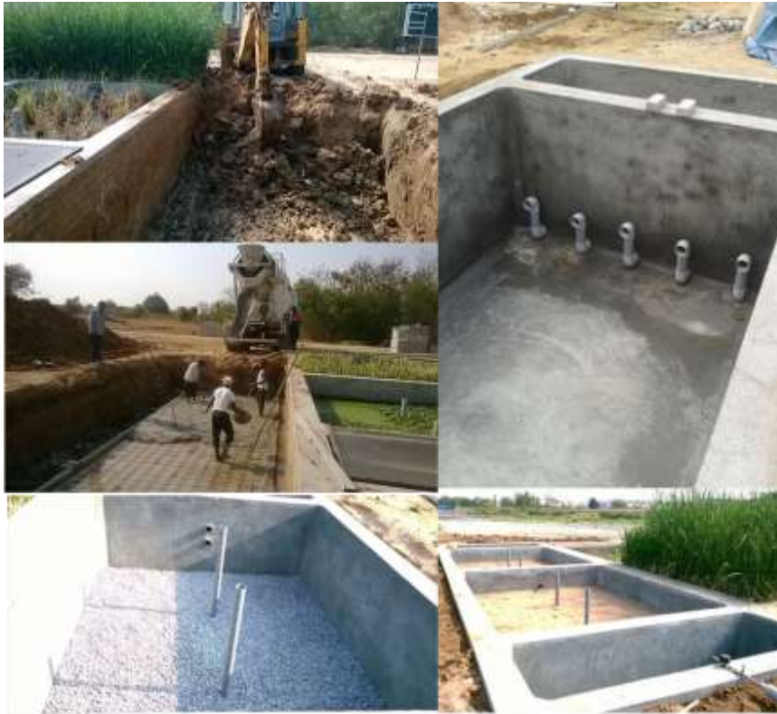
Figure 2-13. Phases of new cell construction at the constructed wetlands at ICRISAT, Patancheru
