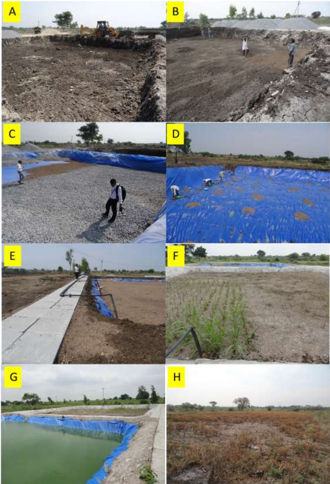
Figure 1-1. Different phases of construction of CW at Sangareddy : A) Excavation; B) Compacting; C) Layering of media; D) Liner in holding tank; E) Pipe fittings at the inlet side; F) Plantation; G) Stabilizing phase; H) Safflower fields irrigated with treated wastewater
