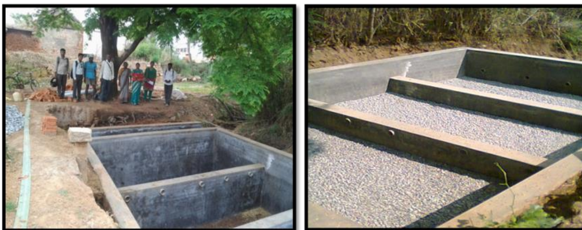
Figure 31. Constructed wetland for domestic wastewater treatment in Mudavatti village, Kolar
