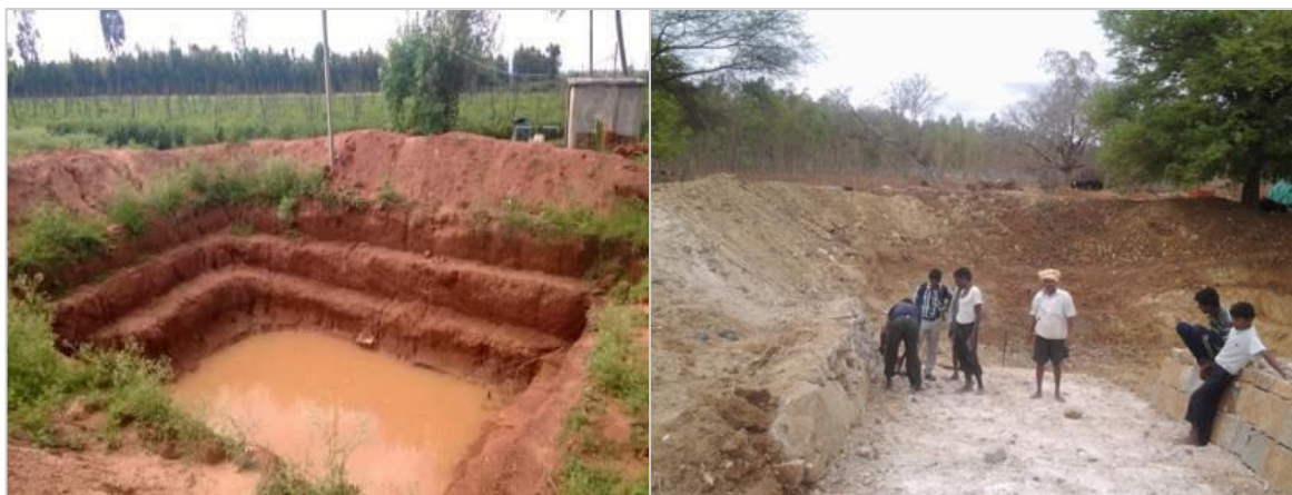
Figure 29. Pictures showing farm pond and Gokatte (percolation tank) constructed at different locations in watershed for rainwater harvesting during monsoon period
