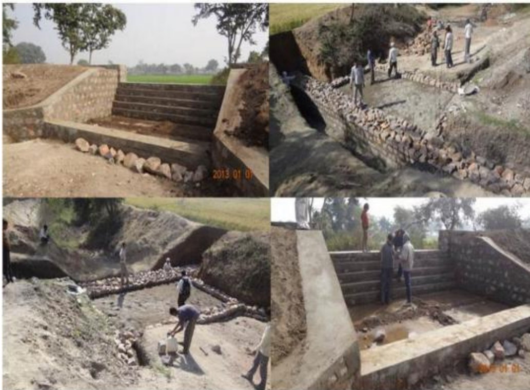
Figure 6. Check dams constructed at different locations in the watershed for rainwater harvesting during monsoon period
