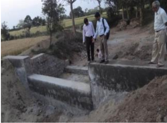
Constructed checkdam under project
