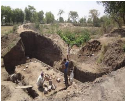
RWH structure (checkdam) under construction during 2013
