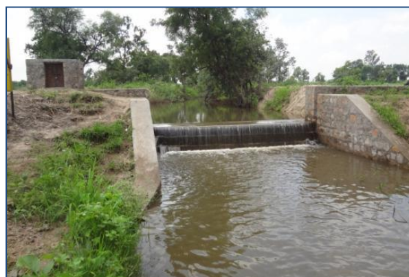
Figure 28. Runoff monitoring system installed at different checkdam locations (logger installed in locked room at left corner of the picture).
