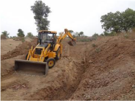
Deepening in the upstream of RWHS constructed during 2012
