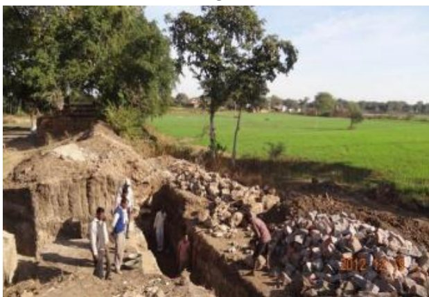
Haveli (Traditional RWHS) outlet under construction
