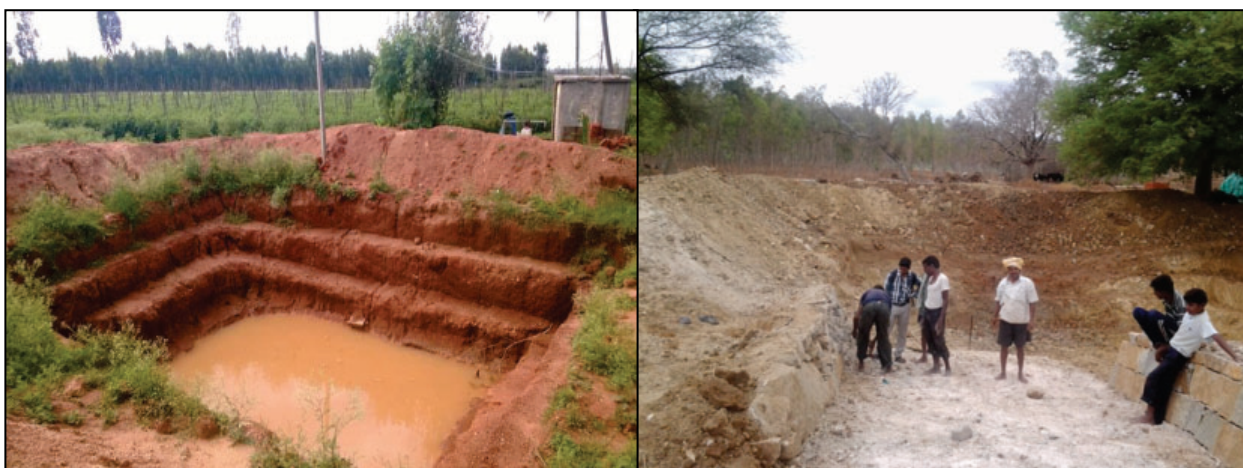
Figure 7. Pictures showing farm pond and Gokatte (percolation tank) constructed at different locations in watershed for rainwater harvesting during monsoon period
