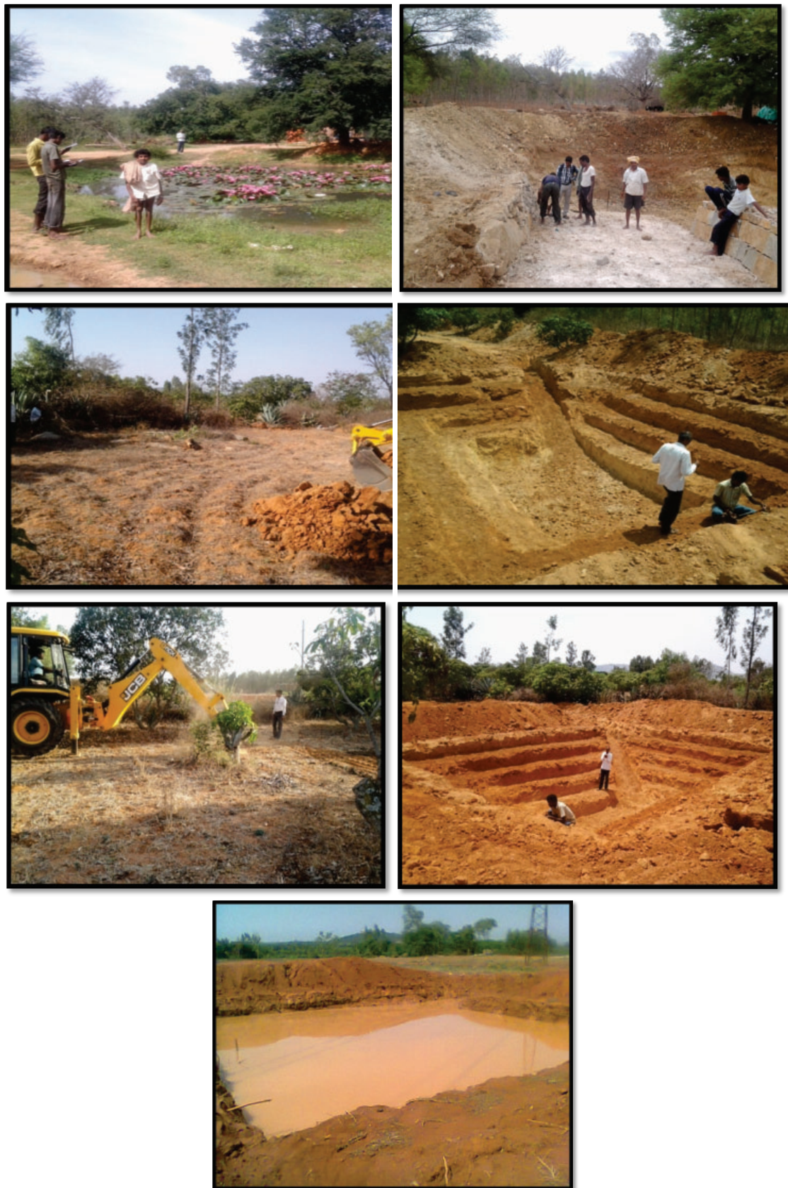
Figure 8. Pictures showing before and after construction of water harvesting structures in different watershed villages in Kolar
